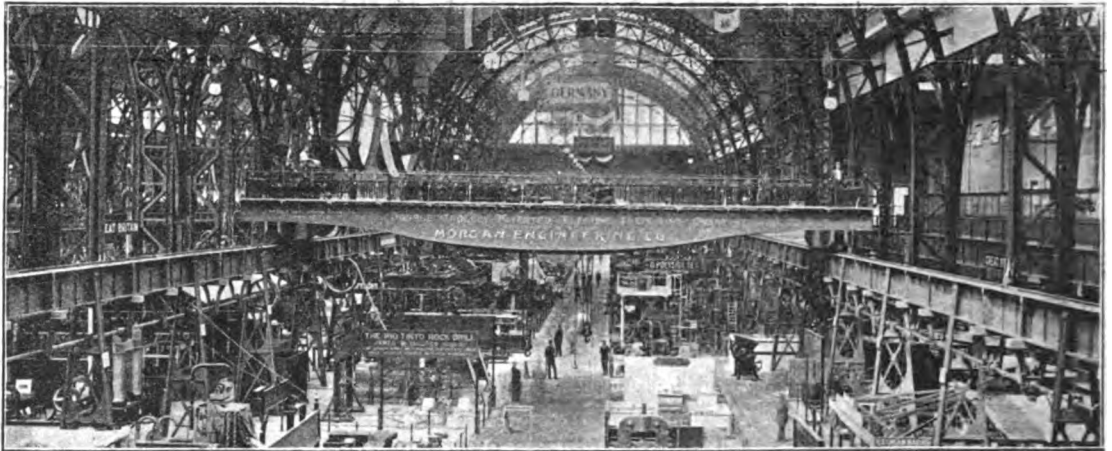
25-Ton Electric Overhead Travelling Crane; Span, 75 Feet; Runways, 1,400 Feet Long. North Wing, Machinery Hall, "WORLD'S FAIR."—Gold Medal Awarded
