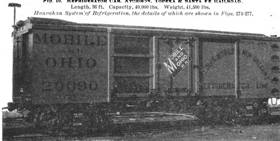
Fig. 11. REFRIGERATOR CAR, MOBILE & OHIO RAILROAD. Capacity, 40,000 lbs. Weight, 37,400 lbs.
