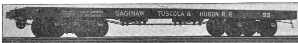
Fig. 16. FLAT CAR. SAGINAW, TUSCOLA & HURON RAILROAD. Length, 36 ft. Capacity, 60,000 lbs. Weight, 20,050 lbs. Equipped with Pull up Brake, Aldrich Brake Wheel and Swing Motion Diamond Trucks.
