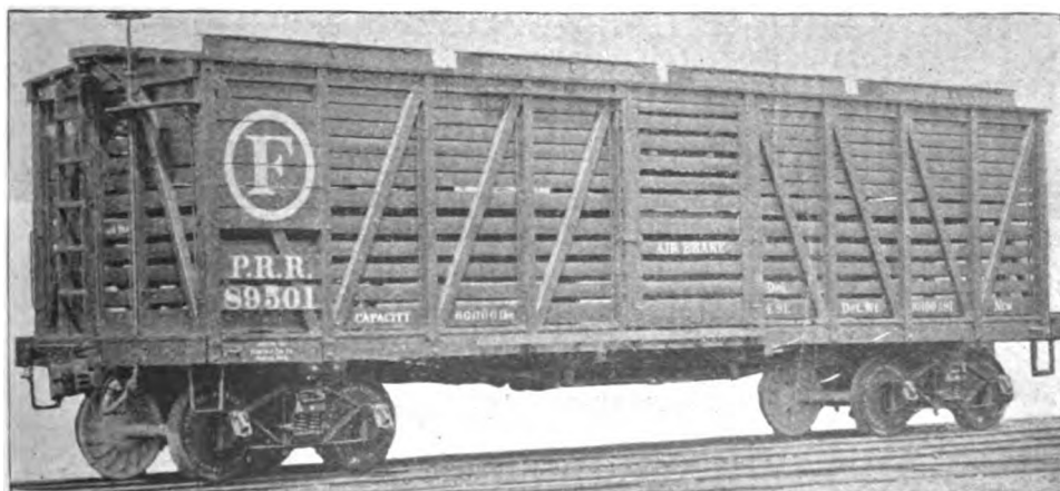
Fig. 38. STOCK CAR FOR CATTLE AND HORSES. PENNSYLVANIA RAILROAD. Capacity, 60,000 lbs. Weight, 30,100 lbs. Equipped with Feed Boxes, Air Brakes and Rigid Diamond Trucks.
